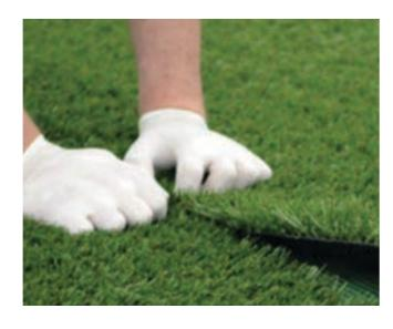
TIP: Brush the grass fibres up where two rolls join to ensure a neat join. Reposition until you are happy with the joins across the whole area.
